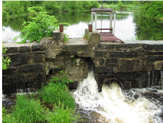
View of the Clary Lake Dam
