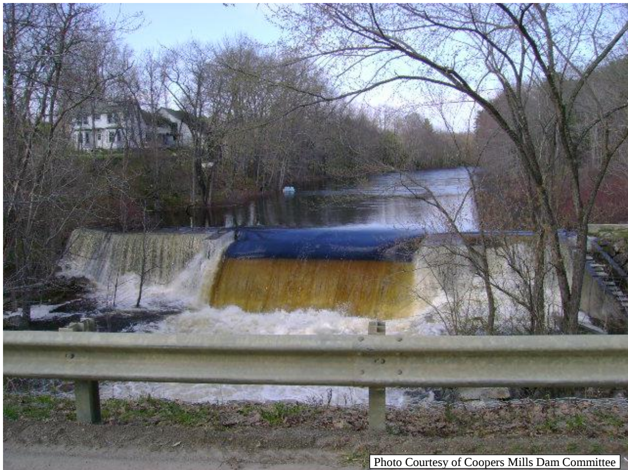
Figure 2. Coopers Mills Dam Overtopping During Spring Runoff, 23 April 2006.
