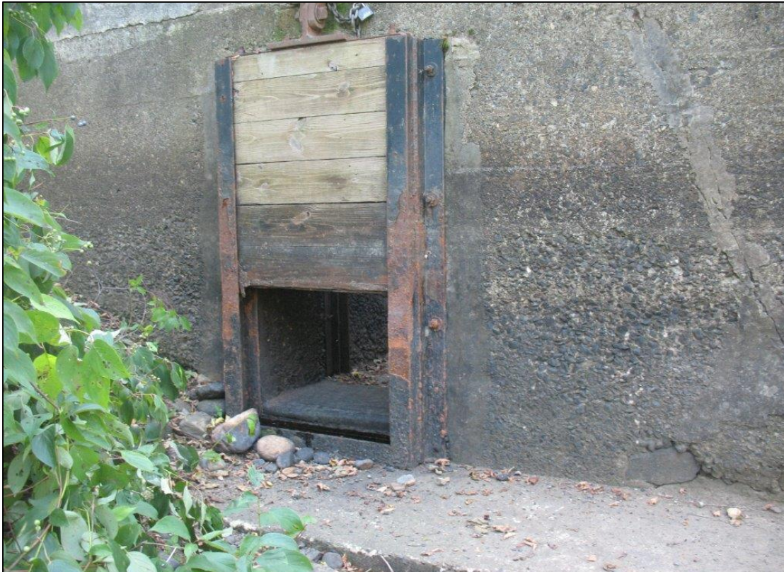
Photo 18. Exposed Upstream Opening and Timber Gate of Fishway.
