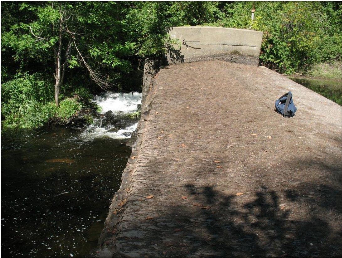
Photo 1. Spillway Crest and Right Pier.
